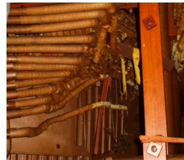
Displaced internal connections
